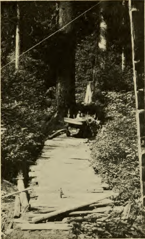
The pathfinder, passing through the giant forest of Snoqualmie Pass, Washington, made his way over atrocious corduroy roads like these, now replaced by an excellent highway
